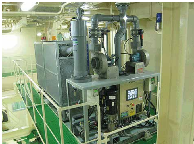
A patented BALPURE seen installed on a vessel
